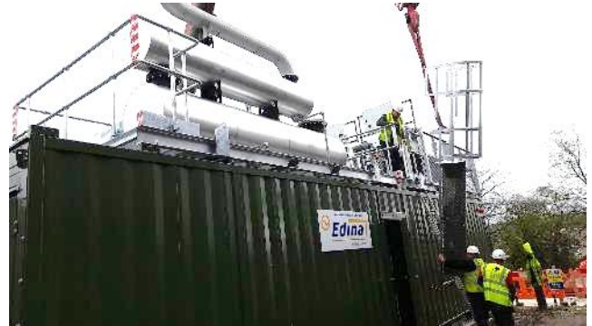
above - Combined Heat and Power Plant install 2023/24 DHH
