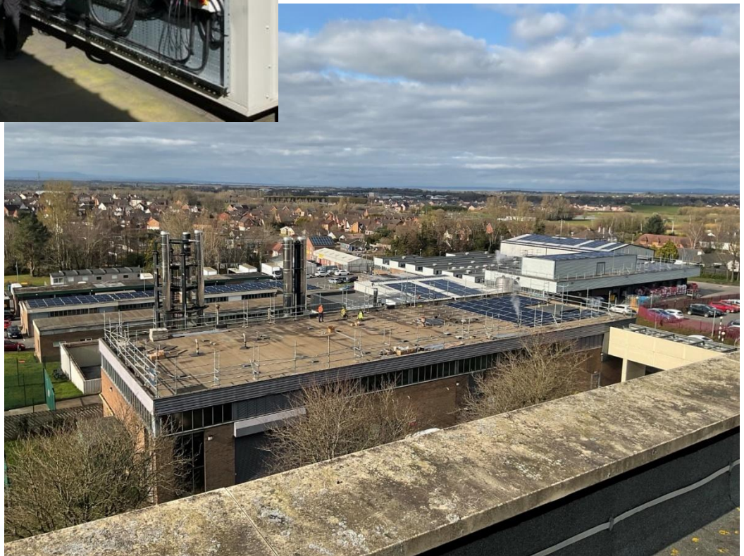
Left and below - Large Scale Solar PV installation on Craigavon Area Hospital 2024/25
