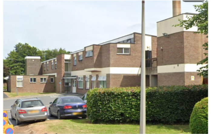
Ashleigh House, St. Luke's Hospital
