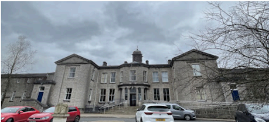
Hollows Building, St. Luke's Hospital
